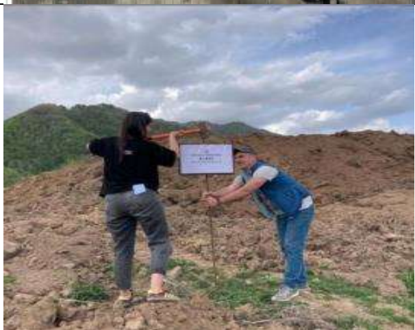
Installation of signs at topsoil storage area April 2024
