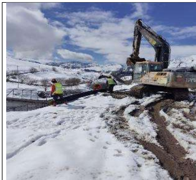
Sedimentation ponds cleaning in Tskere February 2024
