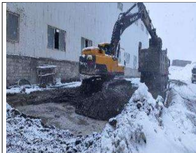
Washout pit cleaning Kobi BP Feb 2024
