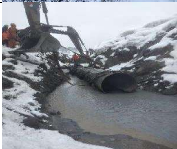
Tunnel water pipe underground being arranged by LOT-1 CC Tskere. March 2024
