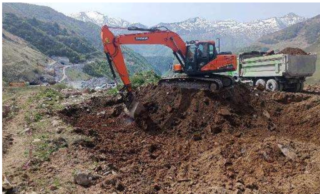
Figure 21: Earthworks near CH 26
