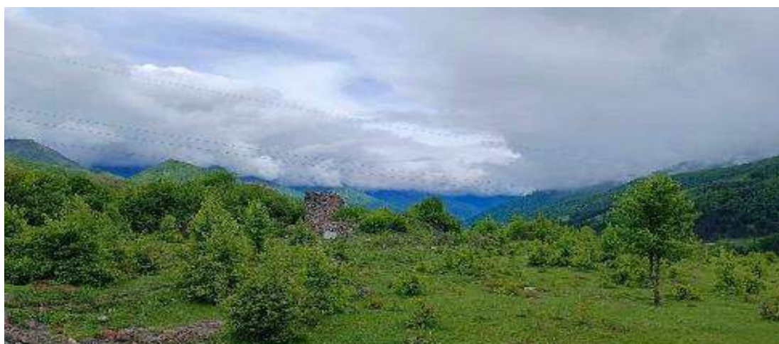
Figure 22: Conservation Works of Didveli Backed Tower (CH Site #10)
