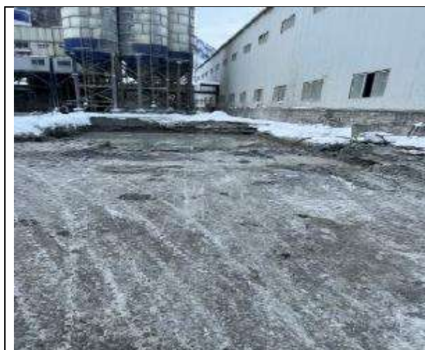
Site cleaning in Kobi batching plant and diesel facility March 2024
